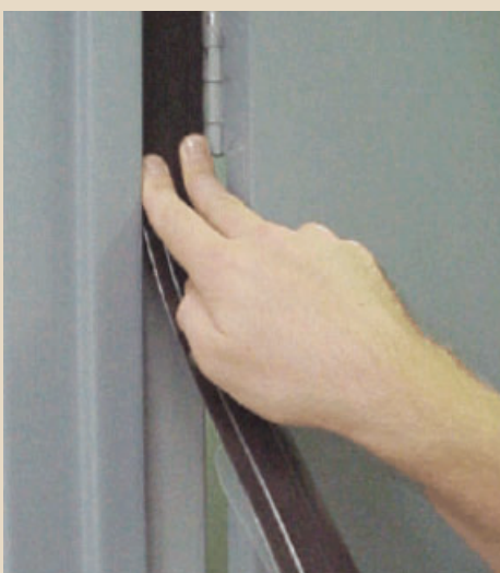
Lorient Australia – HP 4002 product – an example of an self-adhesive type intumescent perimeter seal for use on doors with excessive gaps
