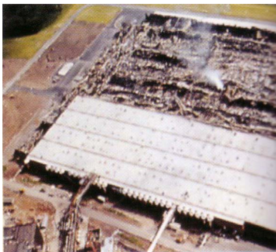
Photo of a brewery fire showing successful compartmentalisation by way of a fire wall
