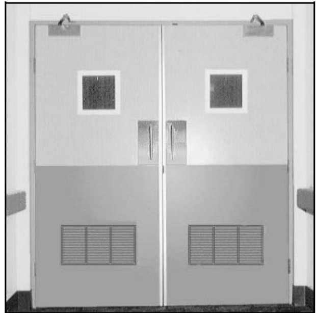
Fire door featuring vision panels and air transfer grilles
