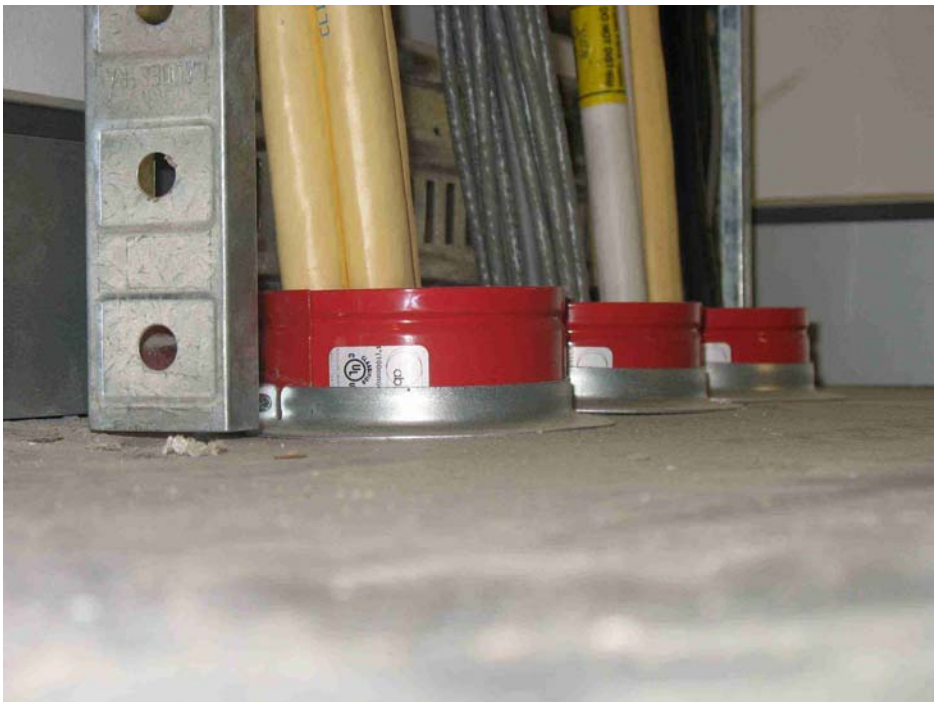
An example of product labeling for identification after installation
